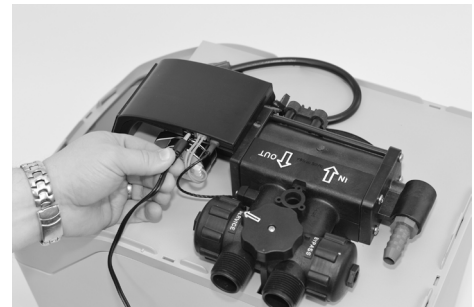
Diagram 15: Connect Transformer Power Cord
